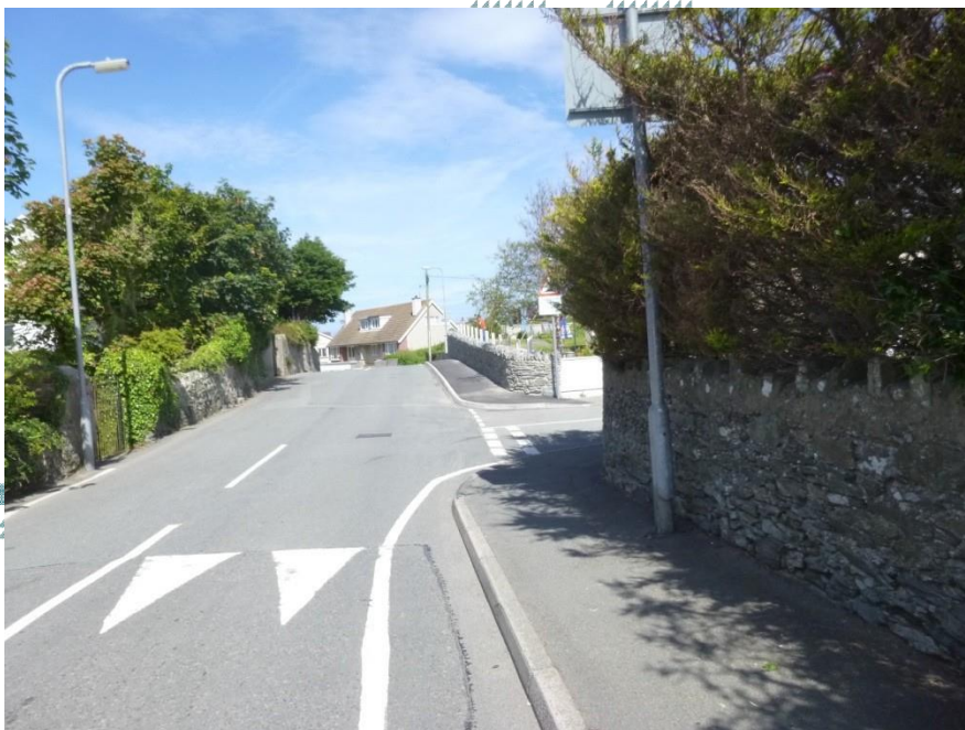
Photograph 7 – Garreglwyd Road west (New footway visible on the right beyond junction to Maes Cybi)
