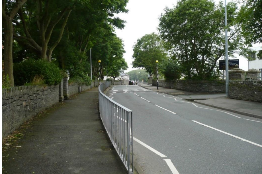
Photograph 1 – View along South Stack Road past proposed site (Site on the left / High School on the right)
