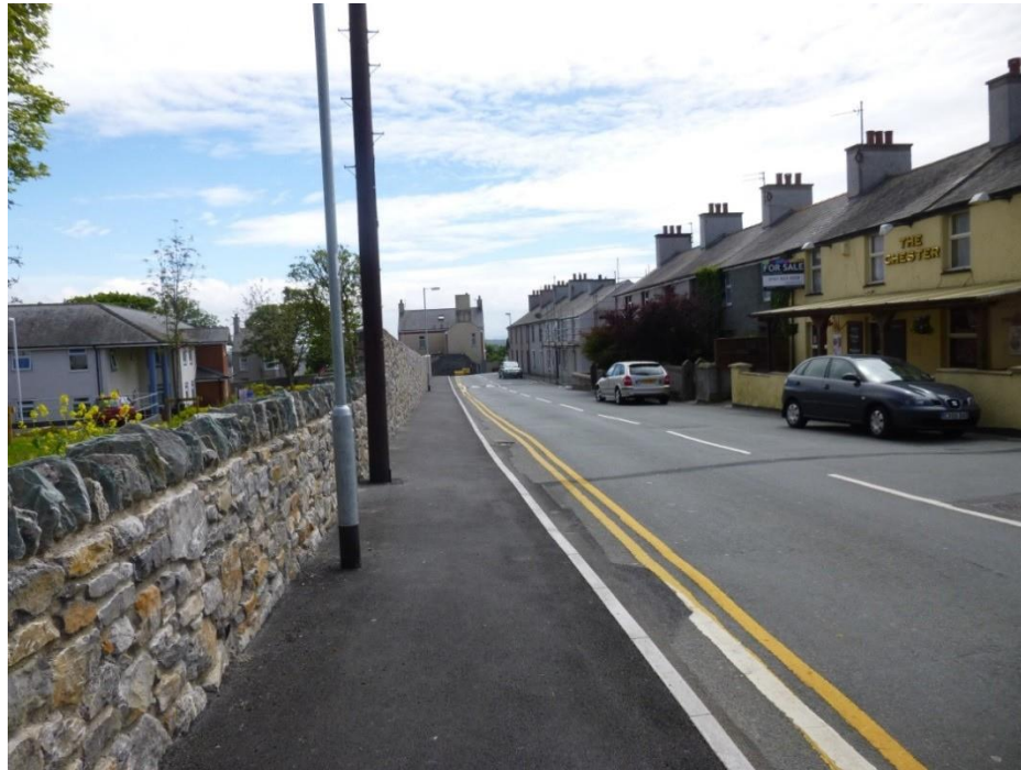
Photograph 8 – New Footway along Mill Bank
