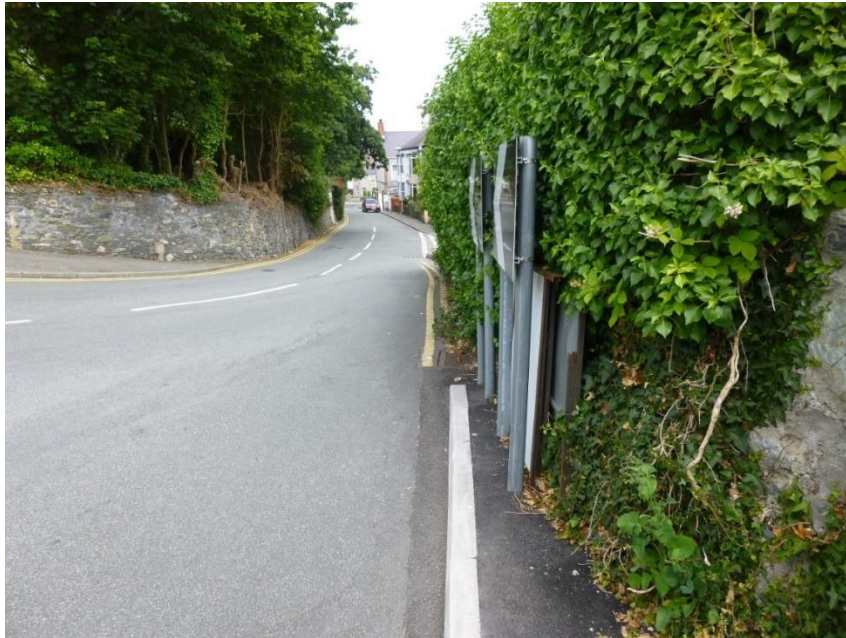
Photograph 18 – Gap in Footway Provision at Plas Road
